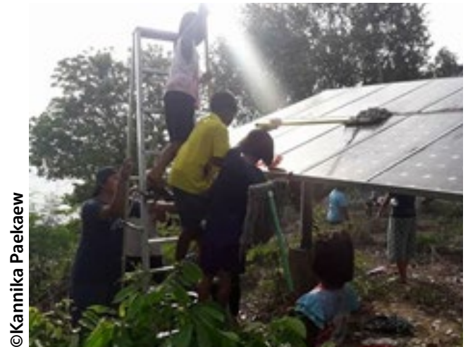
▲ Photo 2.1-6 Volunteers are demonstrating and training on the maintenance of solar panels
