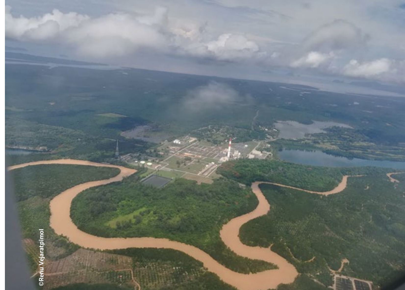
▲ Photo 6.3 Aerial photograph of the Krabi power plant in Nua Khlong District, Krabi Province
