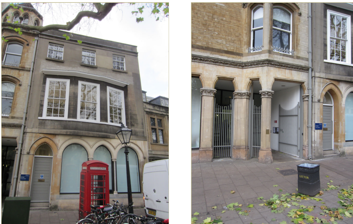
Figure 18. 18.1, left, the bay window of 65 following recent renovations. 18.2, right, the window of 66 converted into the main entrance of the Classics Centre
