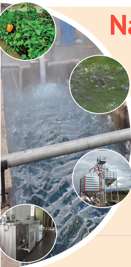
▶ **The geothermal heat exchanger (main) at the Direct Use pilot project at Menengai that is used for (from top) greenhouse heating, aquaculture, grain drying and milk pasteurisation**
