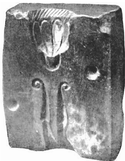
MOULD FOR CASTING ORNAMENTS.
