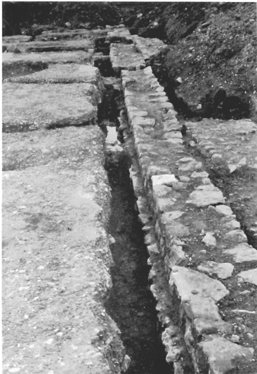
FIG. 14. EAST WALL : PITCHING ON OUTER FACE AND OFF-SET ON INNER FACE ( see p. 342)
